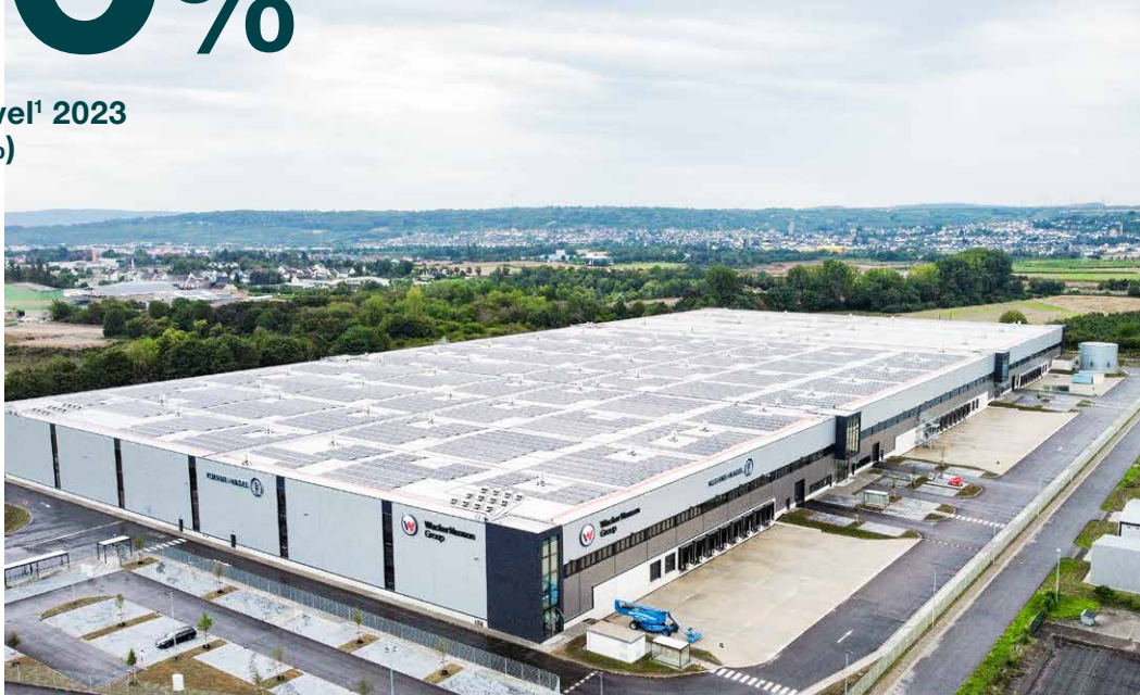
Newly opened in 2023: Mühlheim-Kährlich logistics centre
