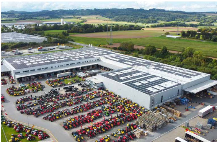
Photovoltaikanlage in Korbach
